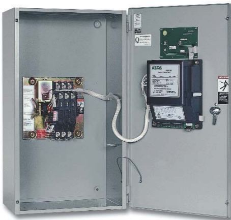
Fig. 2: ASCO Power Transfer Switch rated 200 amperes
