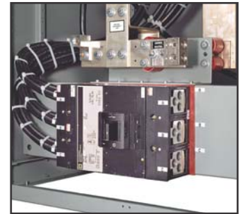
Fig. 16: Ground and neutral disconnect links
