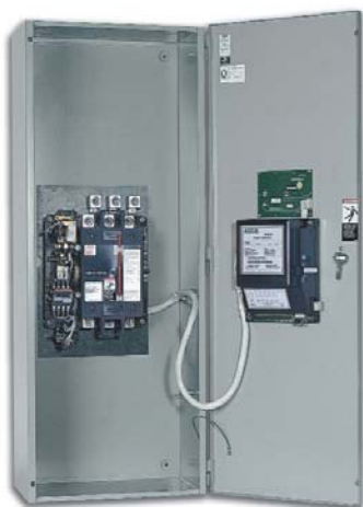
Fig. 3: ASCO Power Transfer Switch rated 400 amperes
